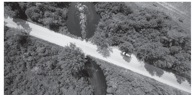
An undersized culvert forms a plunge pool at site #WI-28 (Deer Creek and Fuller Road).
